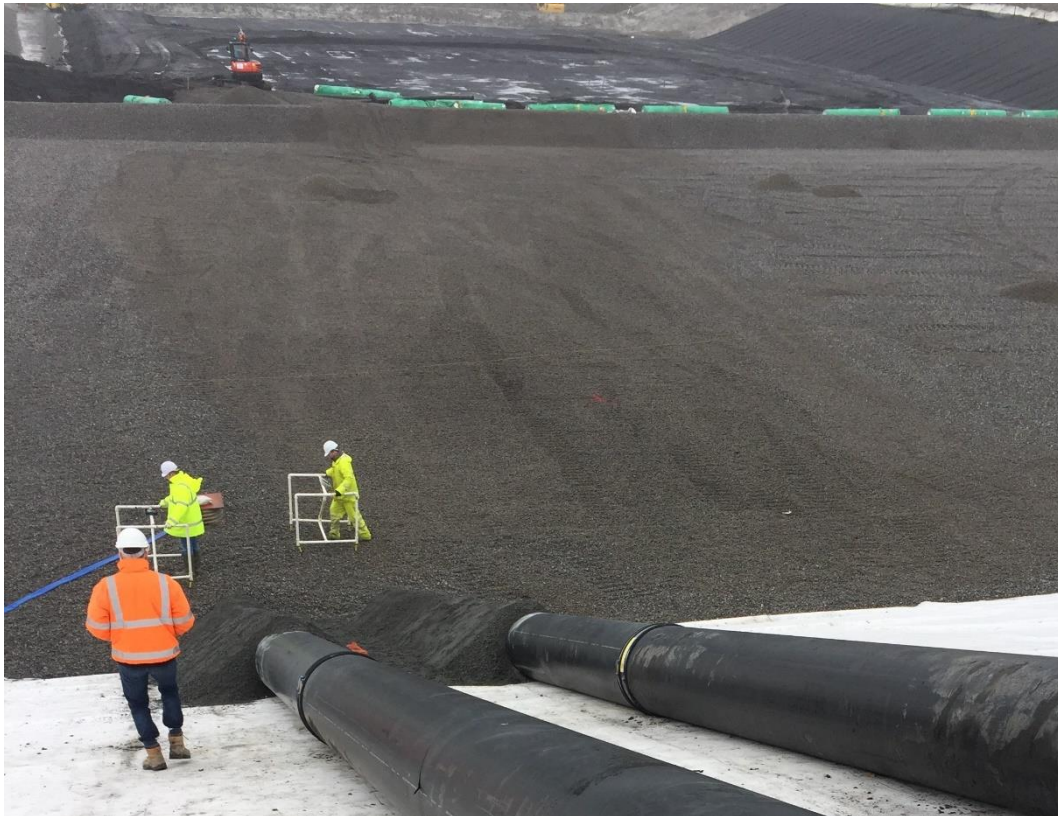
Figure 2-8 – Leak detection test in progress at existing Drehid WMF
