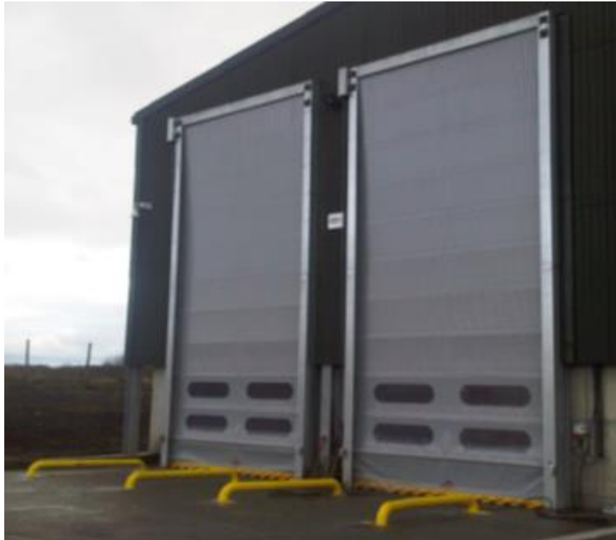
Figure 2-10 – Image of waste receiving doors at existing compost plant
