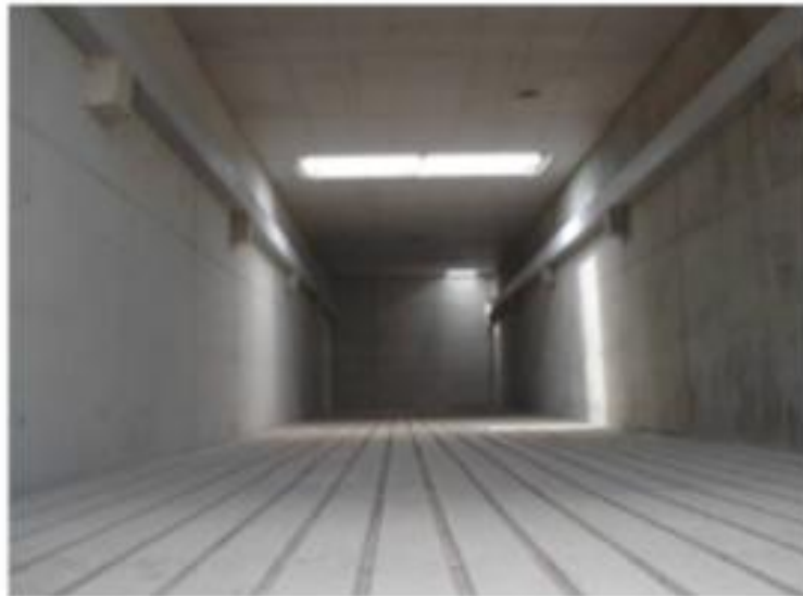
Figure 2-13 - Typical composting tunnel with spigot floor
