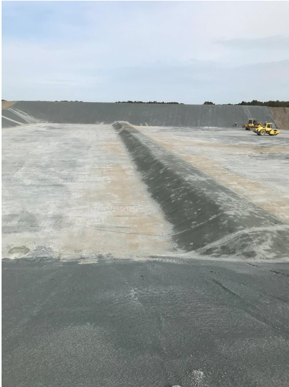
Figure 2-7 – BES liner installed at Drehid WMF
